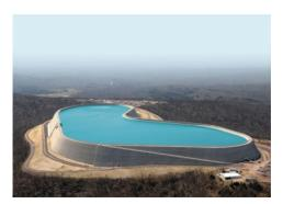
Alstom to construct, operate and maintain Israel's first pumped storage power station in Gilboa - Alstom has signed two contracts totaling around €120 million1 with PSP Investment Ltd for the supply of two 150 MW pump turbines with the associated balance of plant equipment and Alstom's Distributed Control System (DCS) for the 300 MW Gilboa pumped storage power plant in Israel. Alstom also signed an eighteen-year
